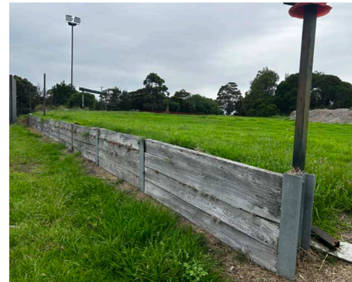
3 Timber retaining wall
