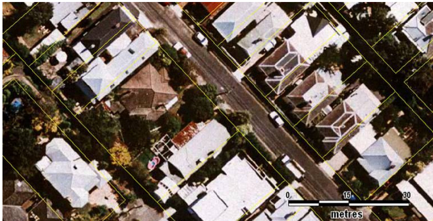
Lawrence Street in the Church Street Centre where the Victorian and Edwardian dwellings have smaller front and side setbacks
