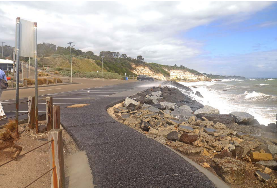
Photo 31: Existing Half Moon Bay car park rock revetment is regularly overtopped
