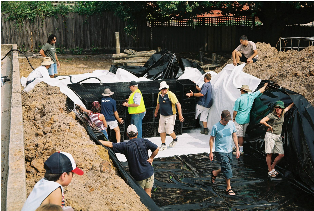
Figure 7: Installation of below ground tank at Hampton Primary School (Source: Bayside City Council)
